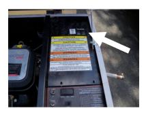
LIFT THE TOP LID OF THE GENERATOR PUSHING DOWN ON THE LID WHILE UNLOCKING (RUBBER GASKET MUST BE DEPRESSED TO HELP EASE THE LOCKING AND UNLOCKING OF LID) TAKE THE ELECTRICAL LOAD OFF BY PULLING BREAKER TOWARDS YOU AND THE FRONT OF THE NEVER DARK GENERATOR.
